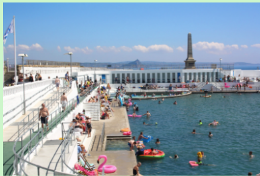
Figure 6. Jubilee Pool geothermal heating scheme, Penzance, Cornwall. Source: (Jubilee Pool, 2018).
