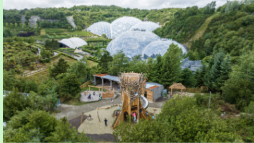
Figure 7. Eden Project geothermal drilling and heating case study. Source: (The Eden Project, 2024) .
