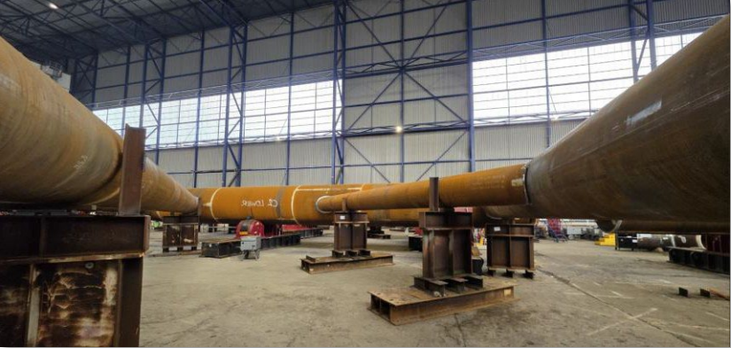
Substation Jacket - Newcastle
