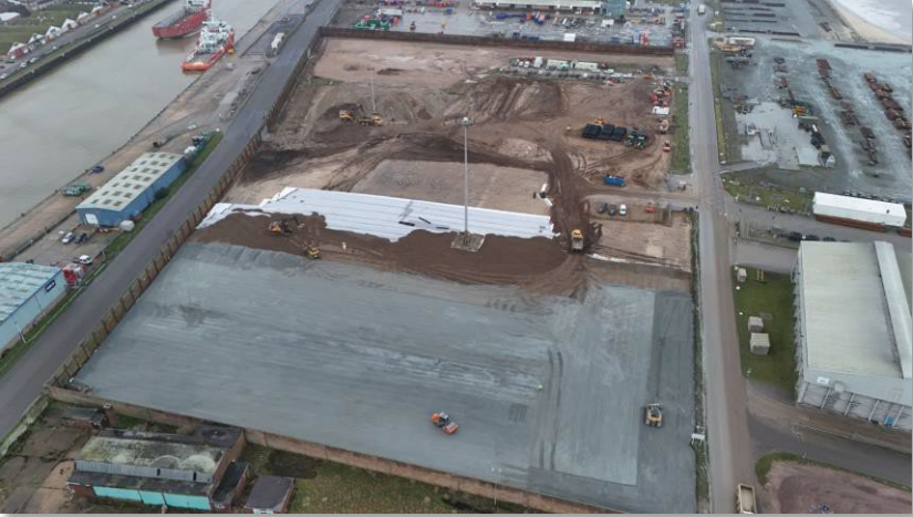
Marshalling Port enabling works - Great Yarmouth
