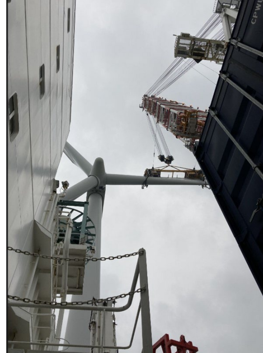
Undertaking turbine maintenance using jack up vessels
