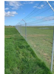
Example predator control fence (Source: Norfolk Projects Offshore Wind Farm, 2022)
